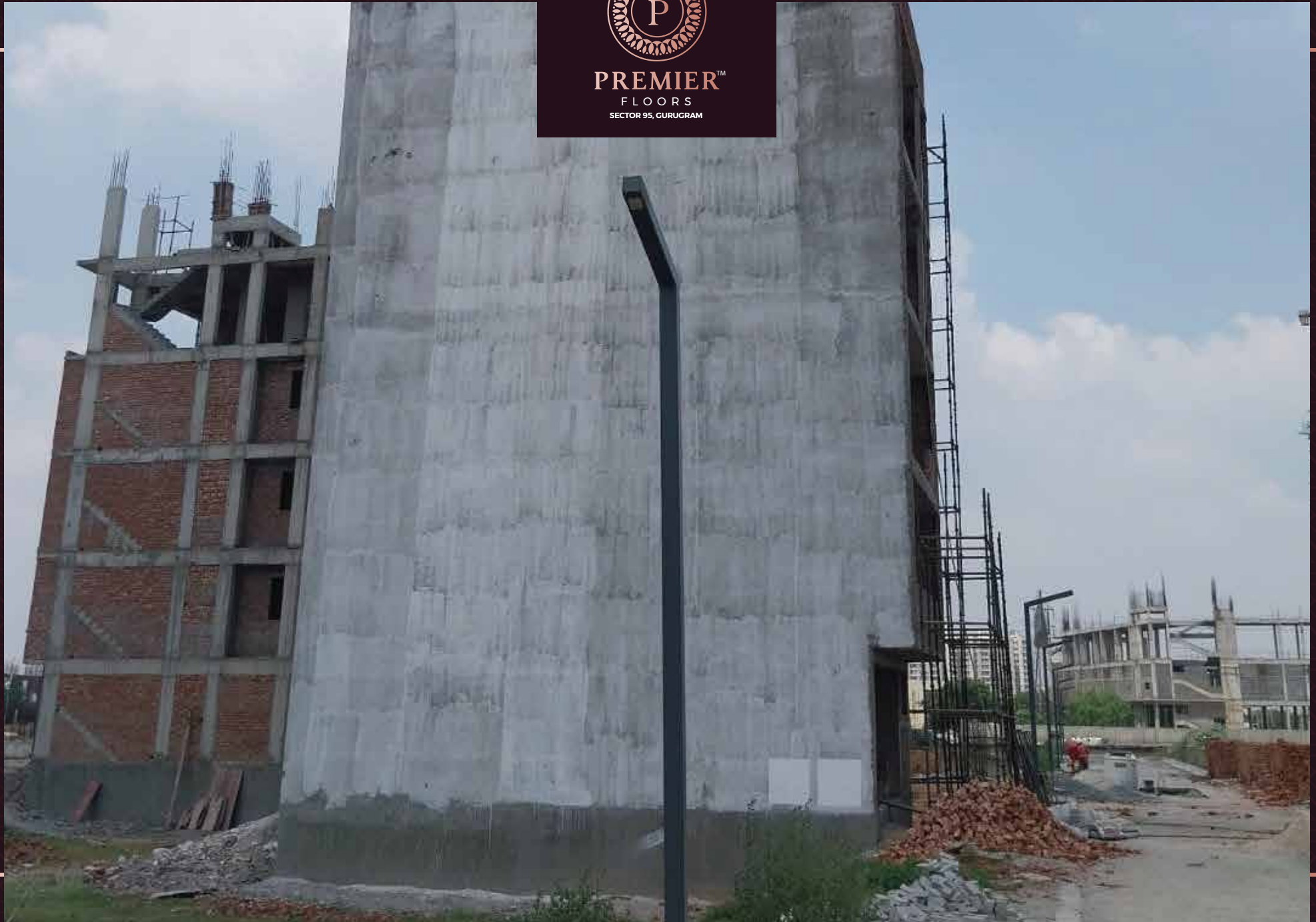
Floors Construction Work In Progress
