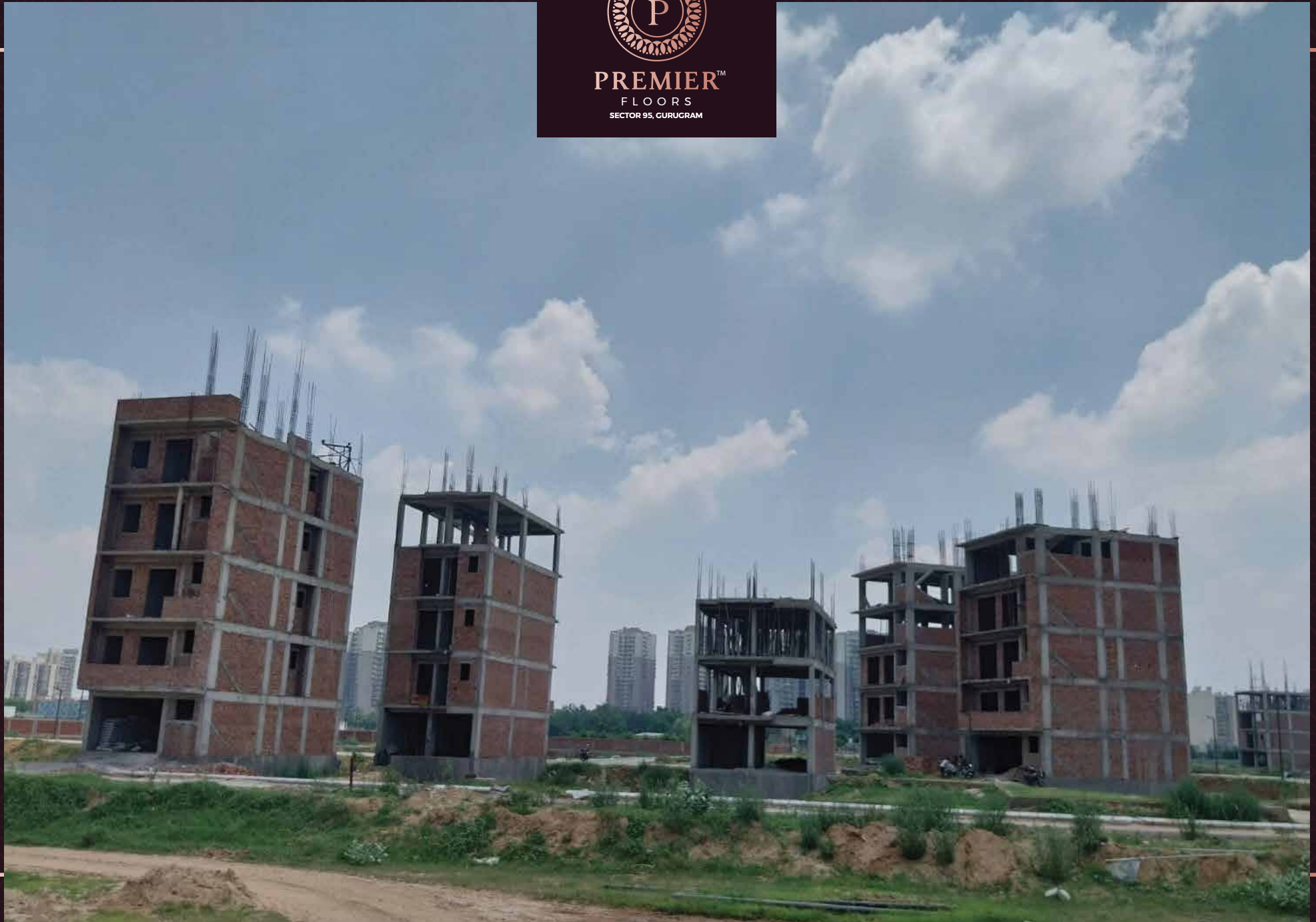
Floors Construction Work In Progress
