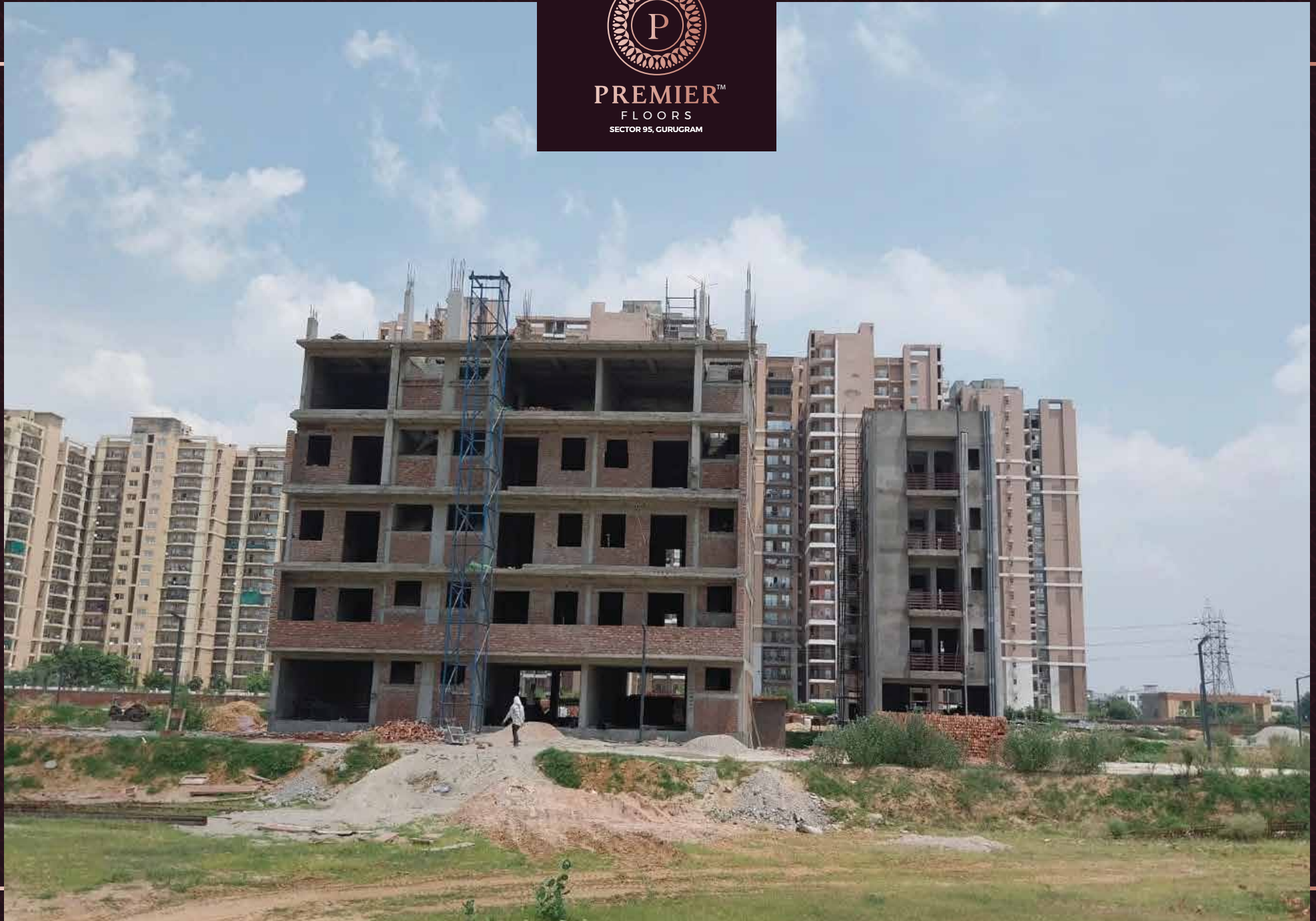
Floors Construction Work In Progress
