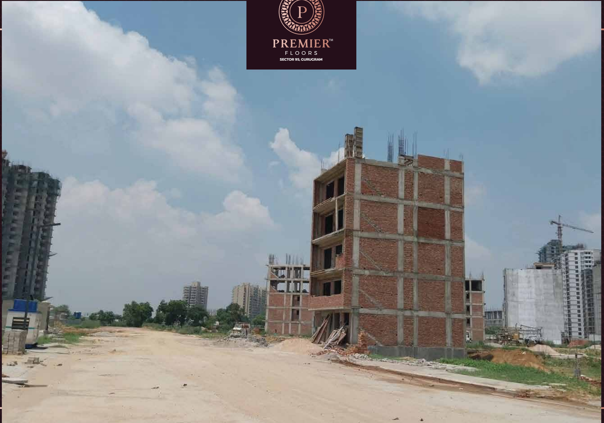
Floors Construction Work In Progress
