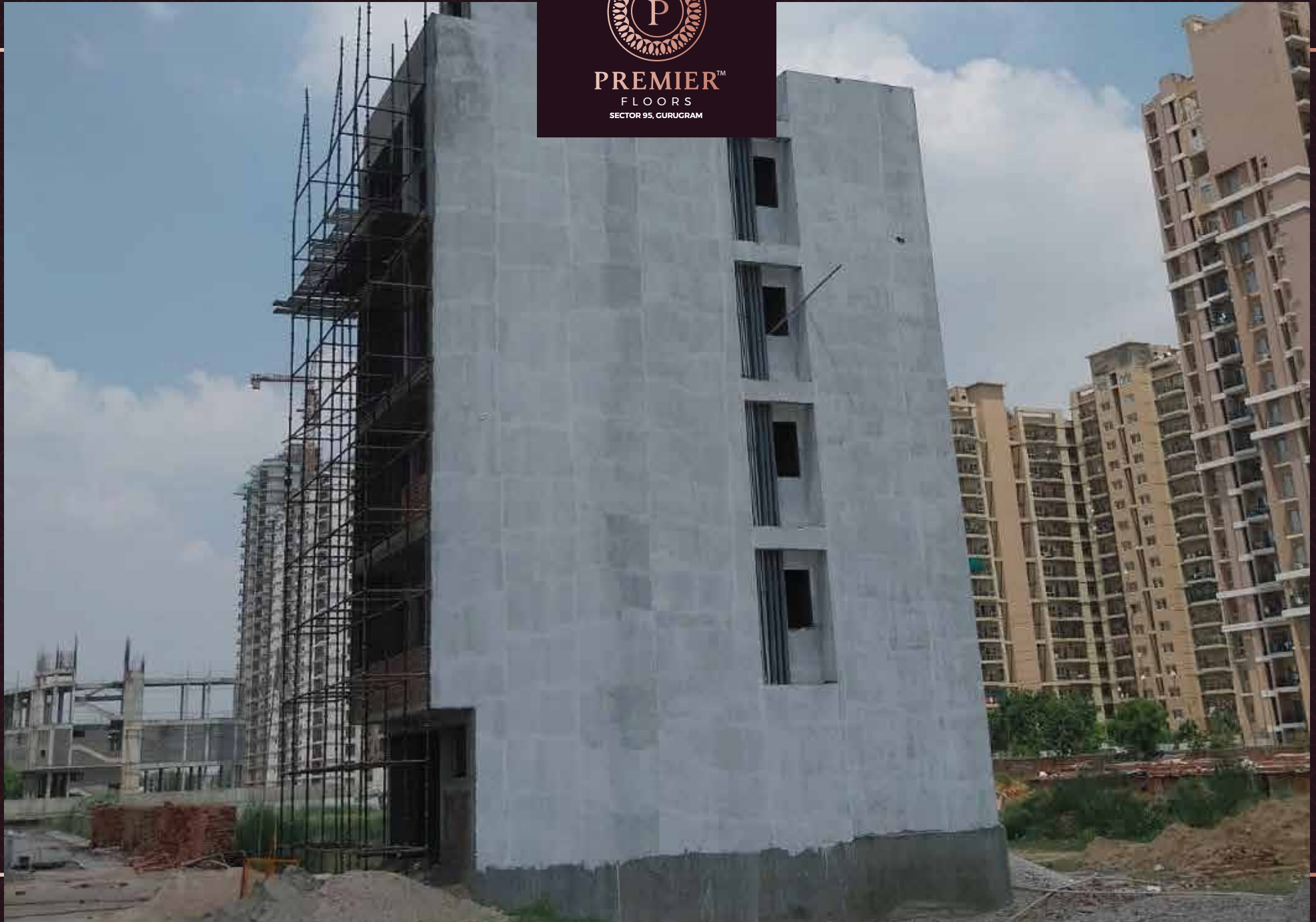
Floors Construction Work In Progress
