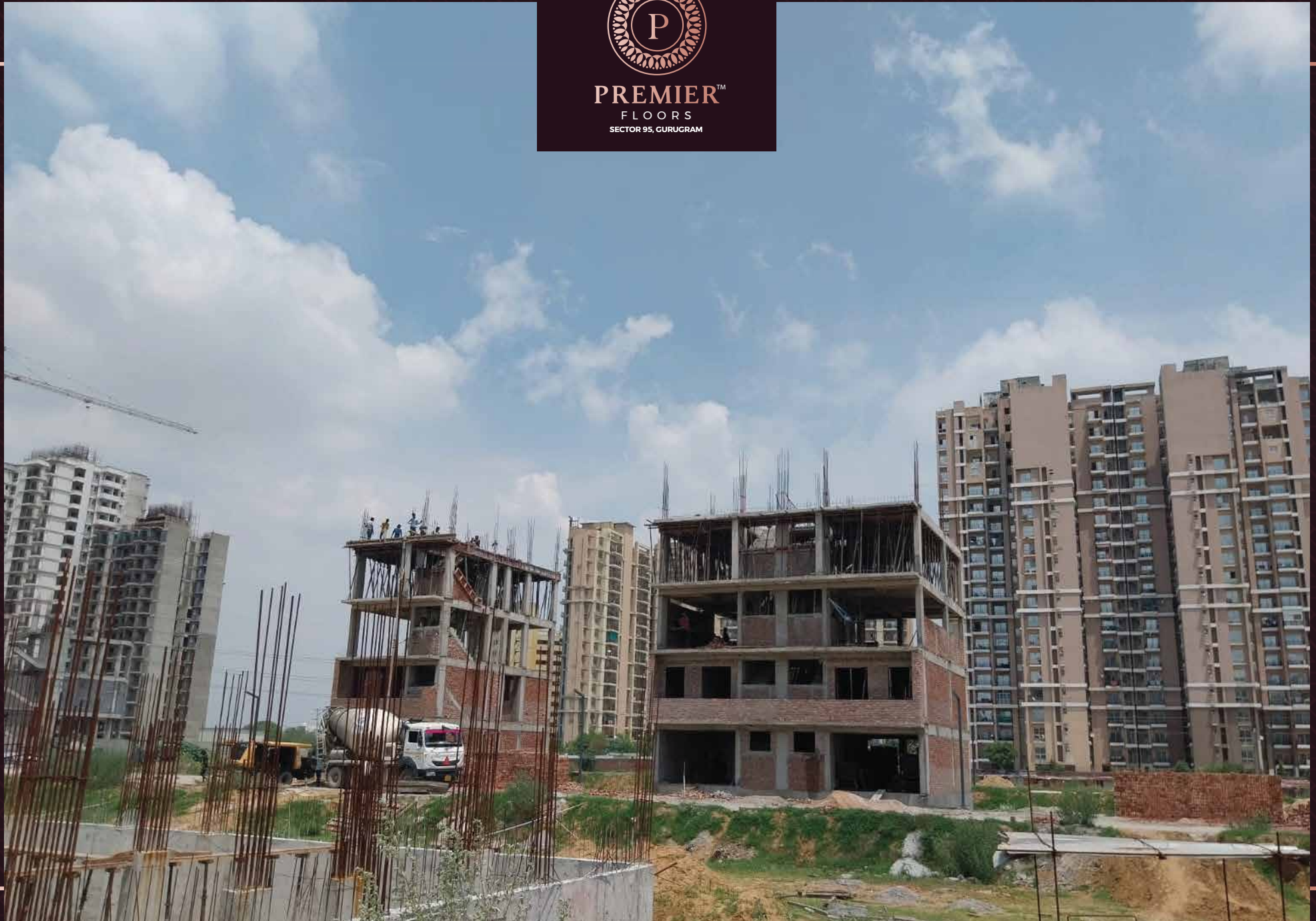
Floors Construction Work In Progress
