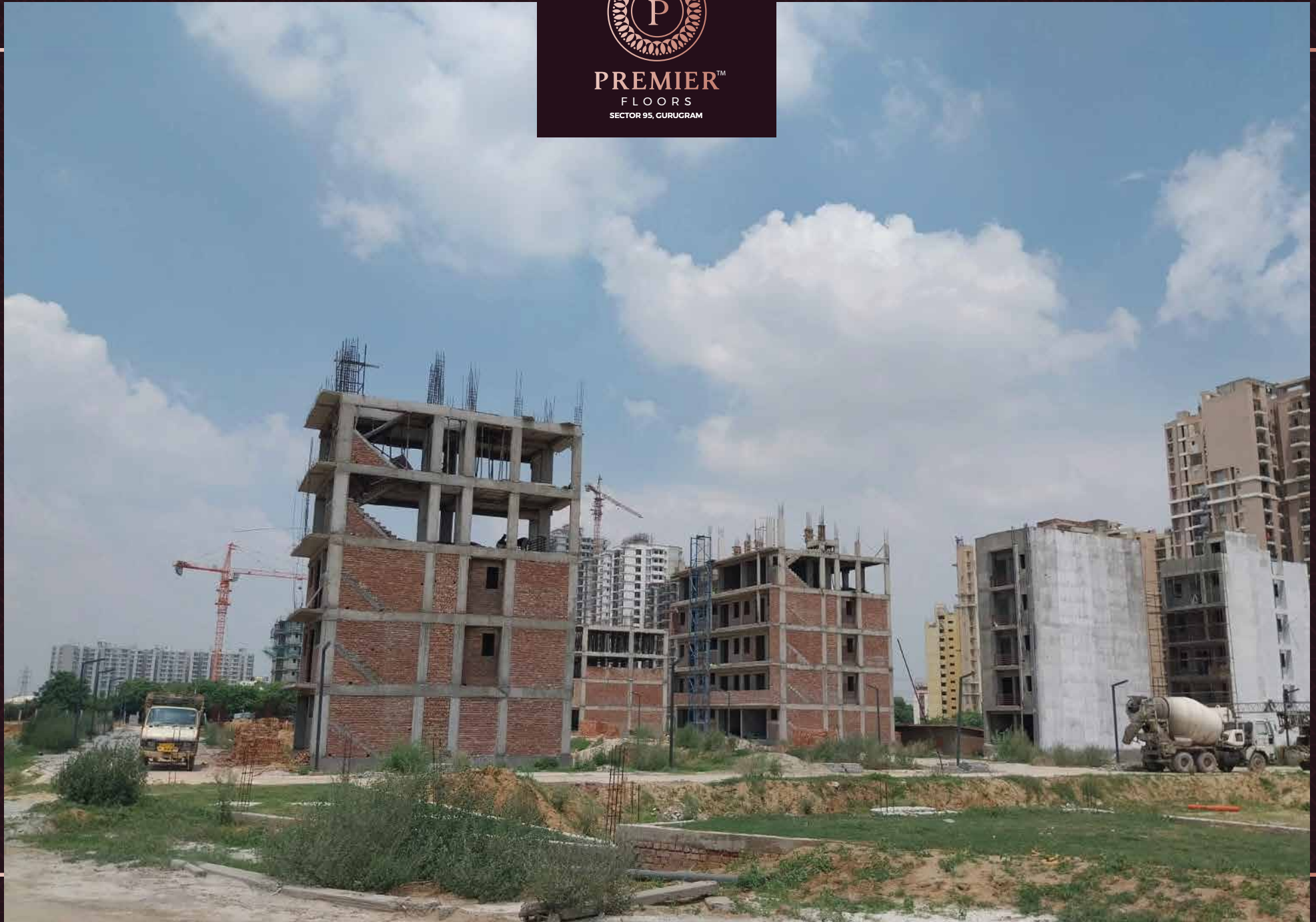
Floors Construction Work In Progress
