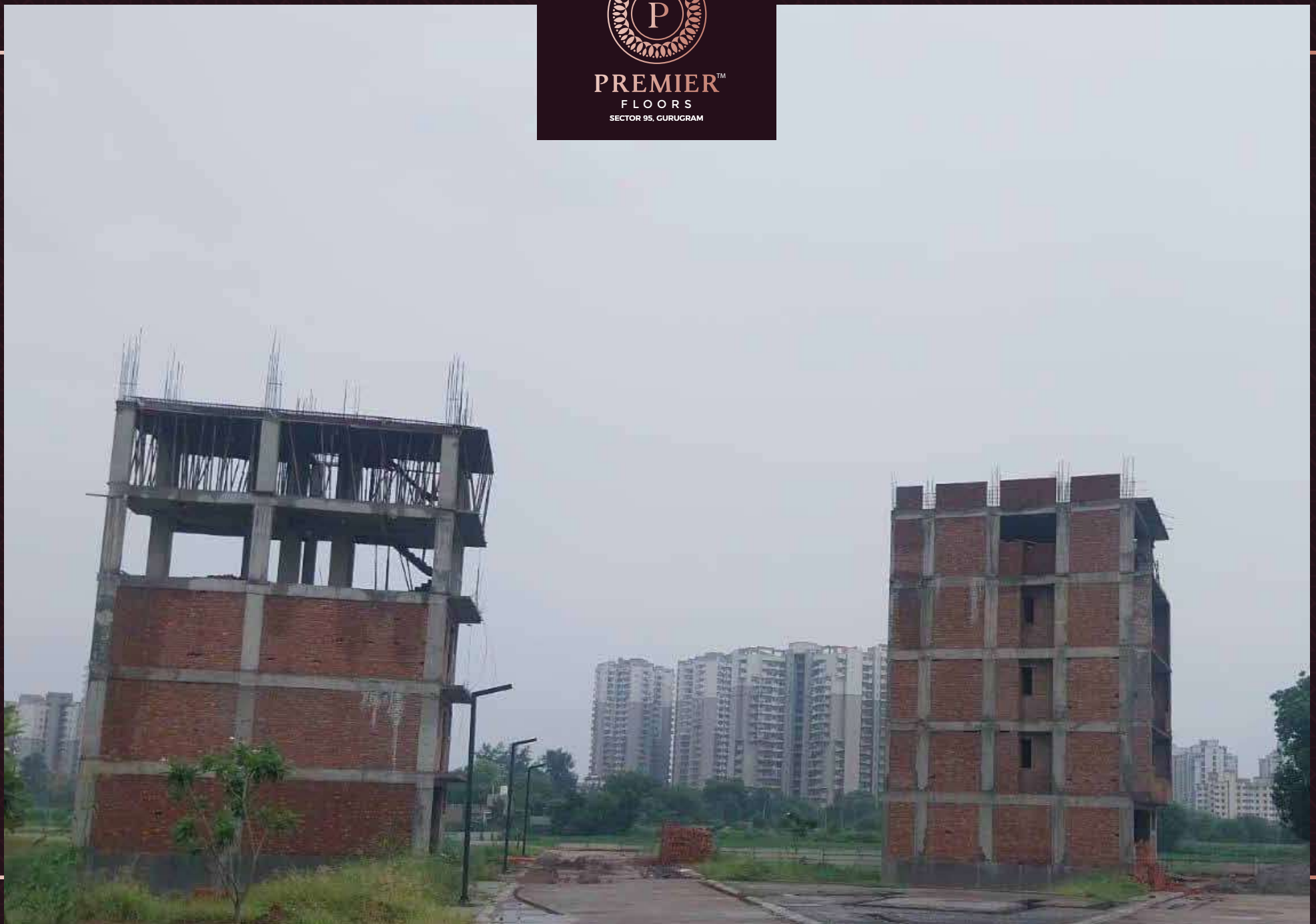
Floors Construction Work In Progress
