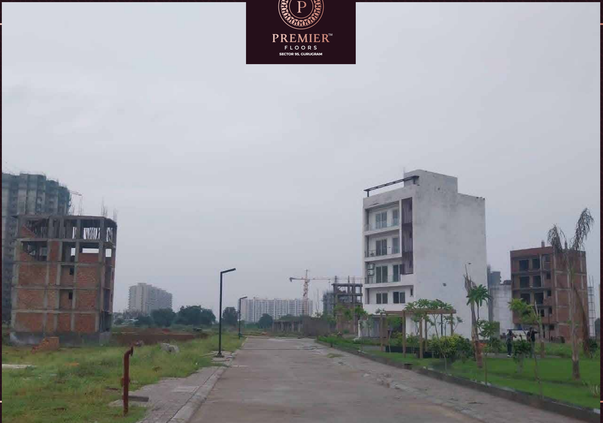
Floors Construction Work In Progress
