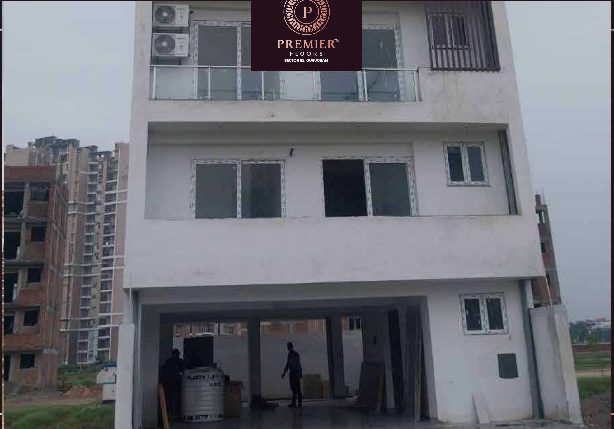
Floors Construction Work In Progress
