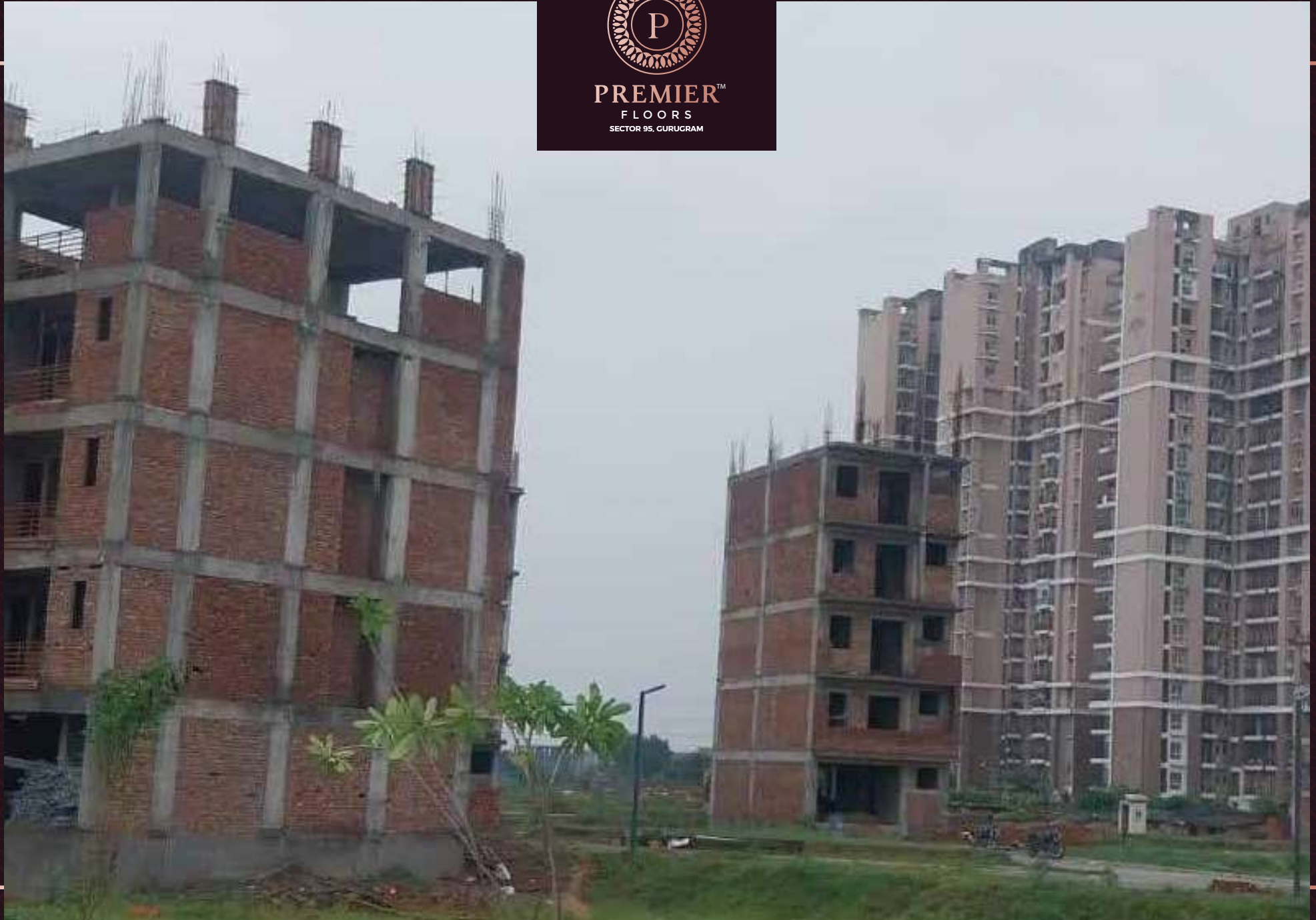
Floors Construction Work In Progress
