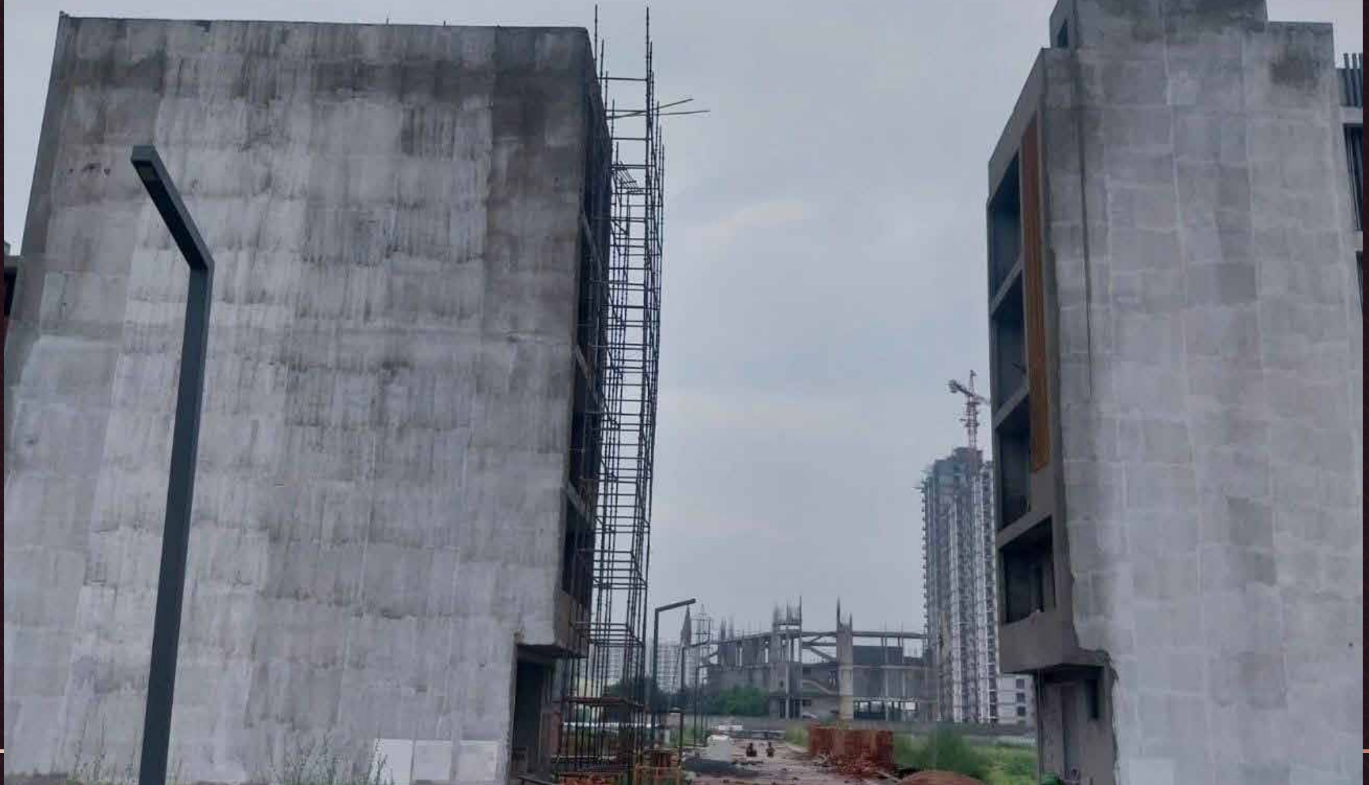
Floors Construction Work In Progress
