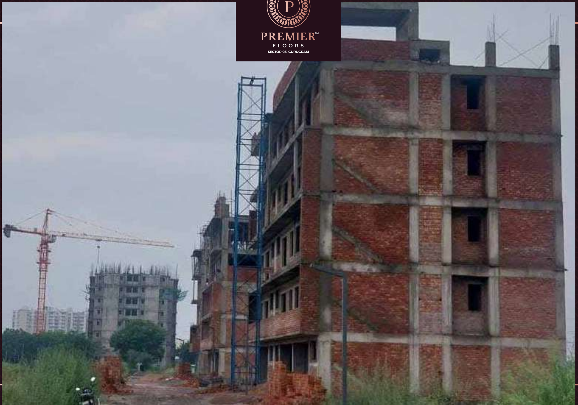
Floors Construction Work In Progress
