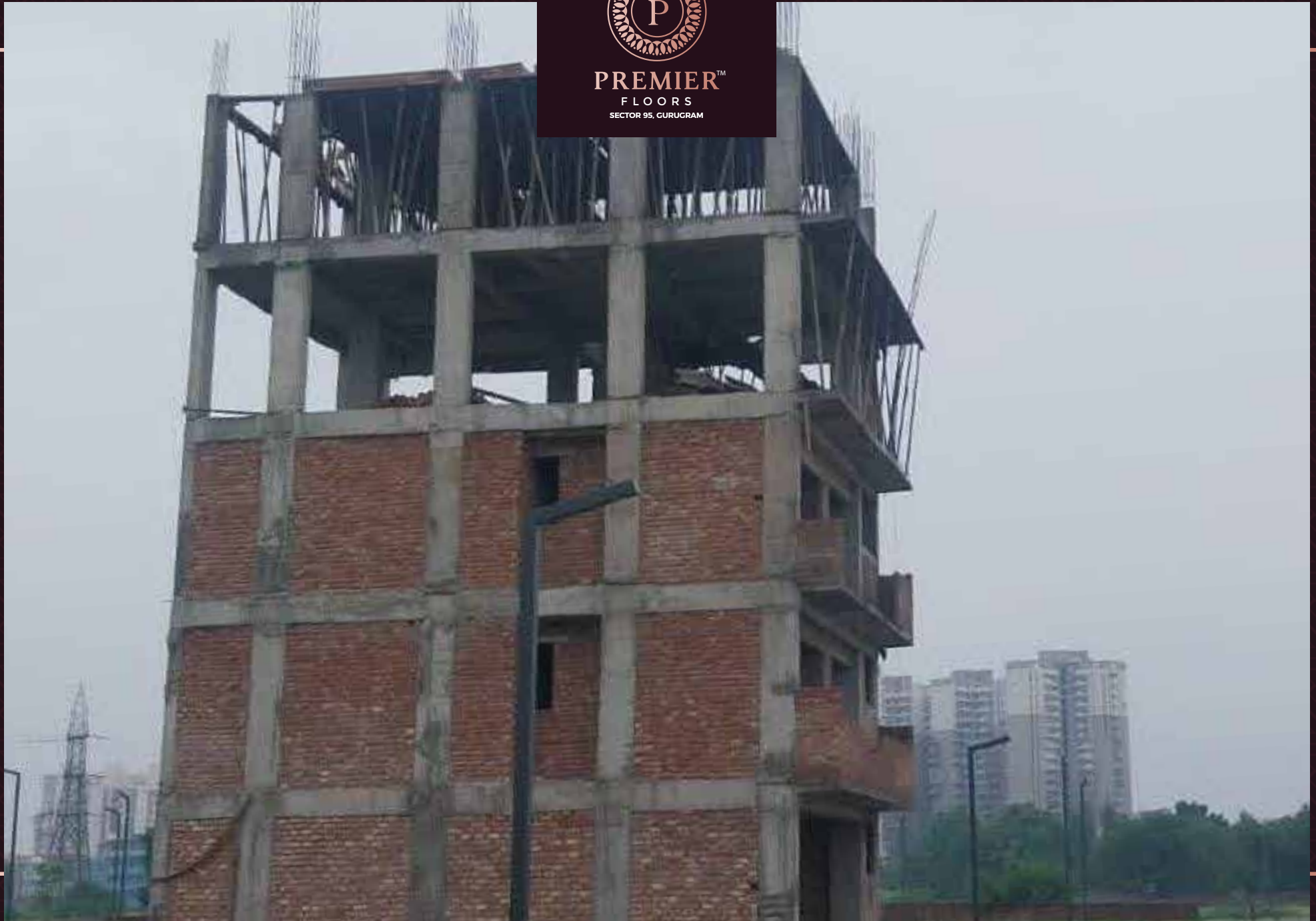
Floors Construction Work In Progress
