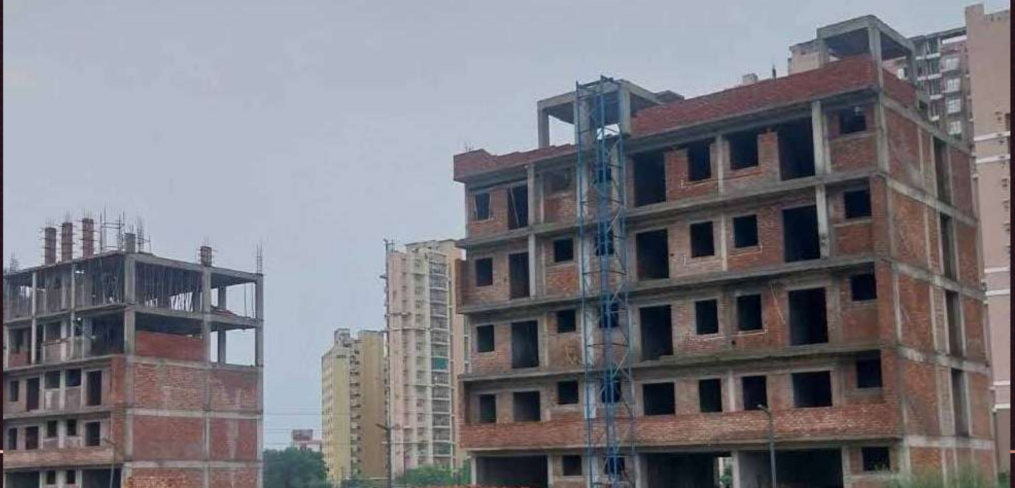
Floors Construction Work In Progress
