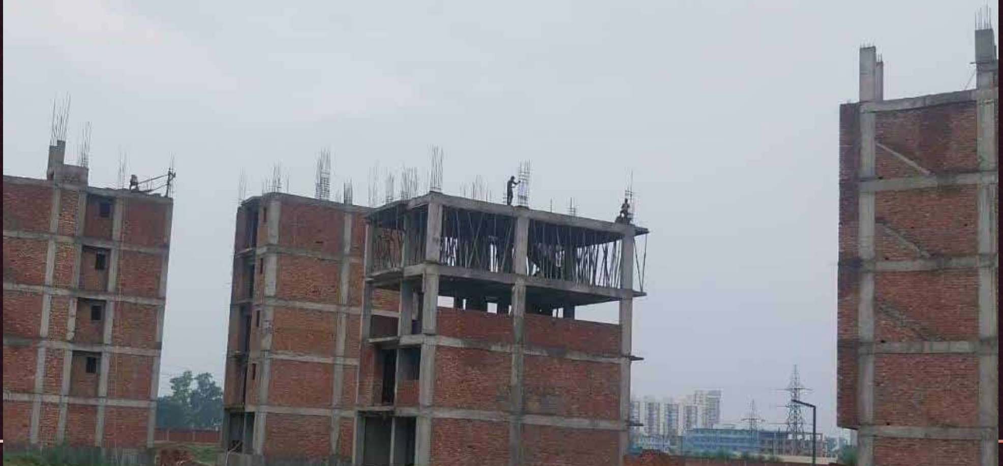
Floors Construction Work In Progress
