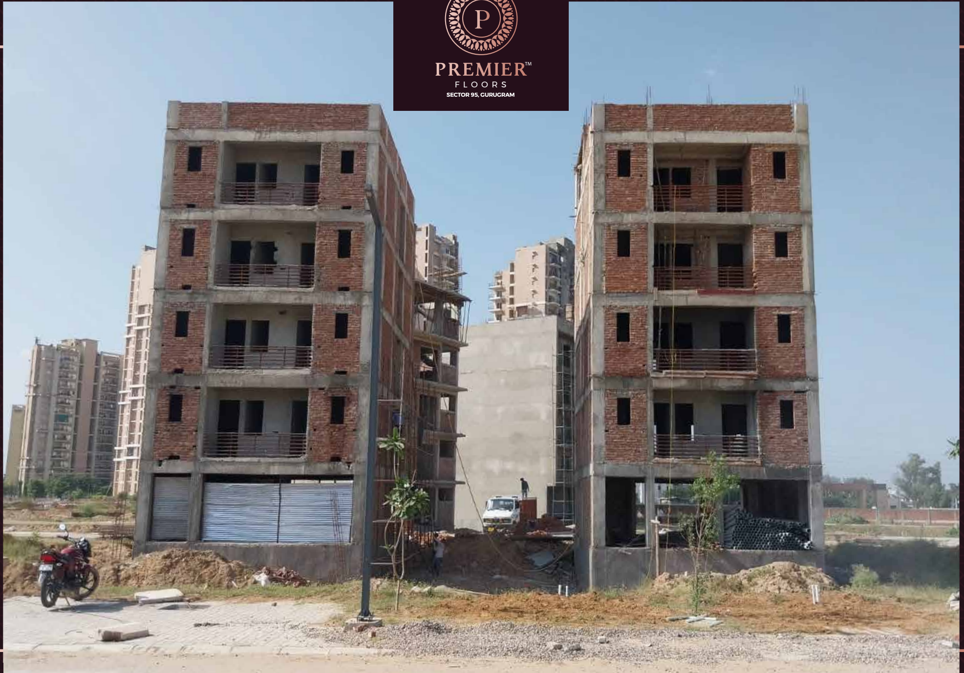
Floors Construction work in progress
