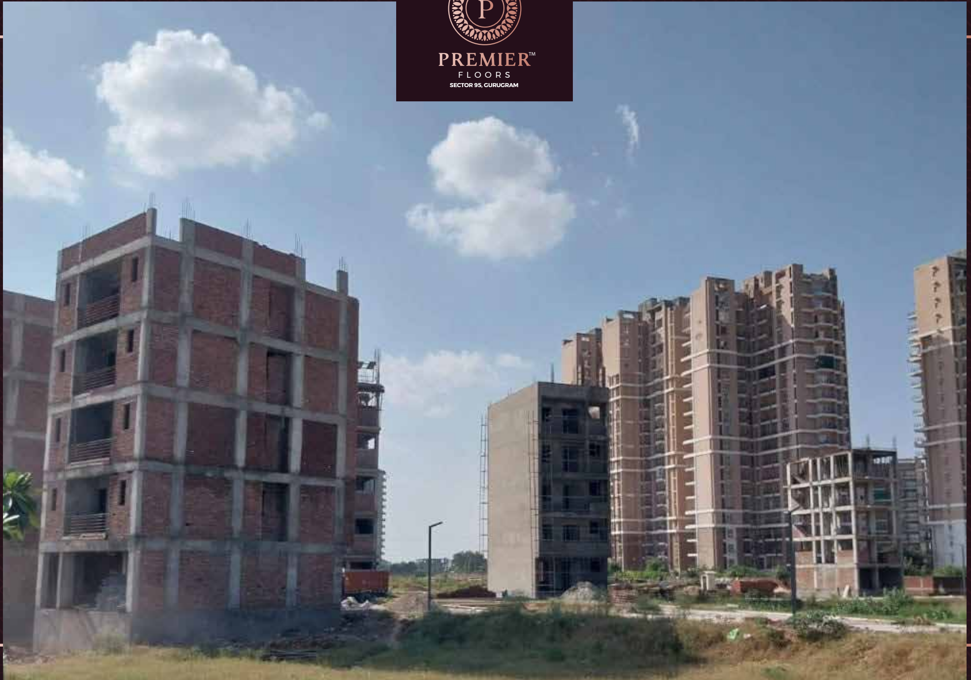
Floors Construction work in progress
