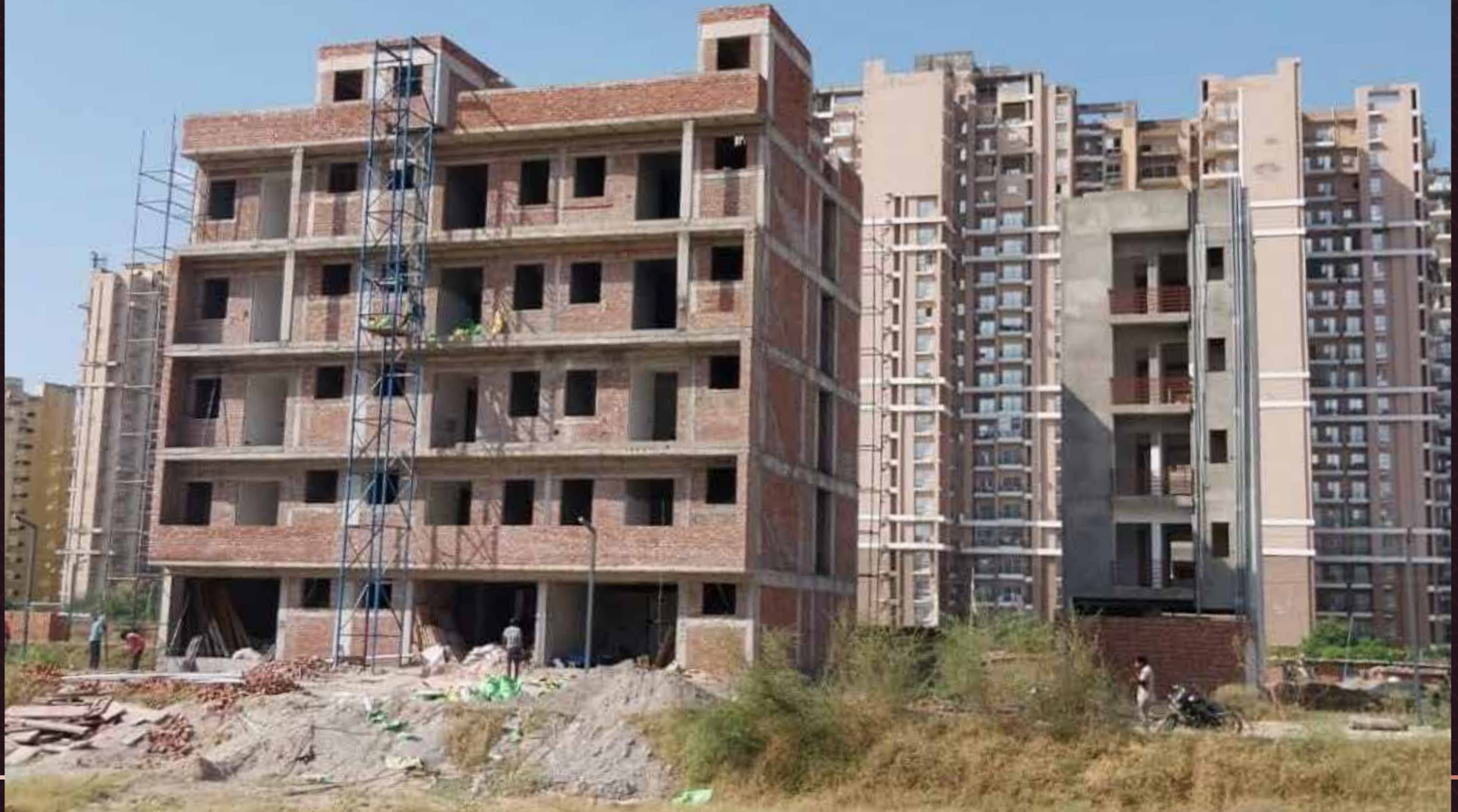
Floors Construction work in progress
