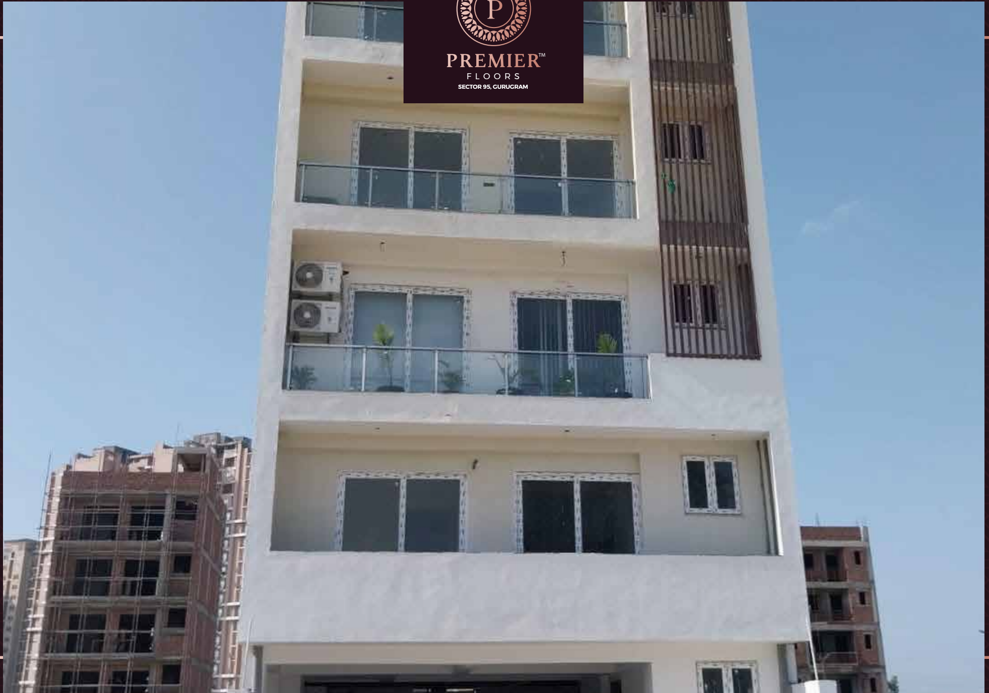
Floors Construction work in progress
