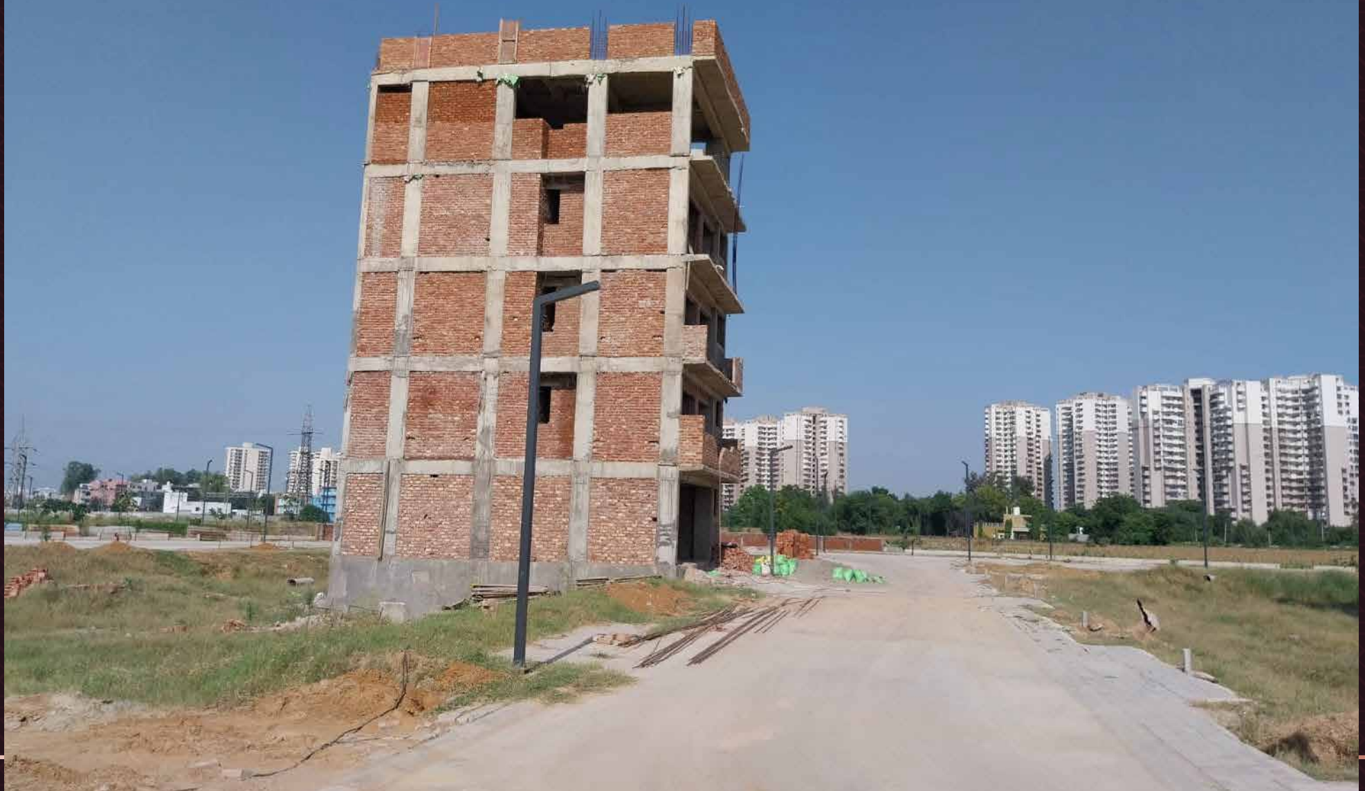
Floors Construction work in progress
